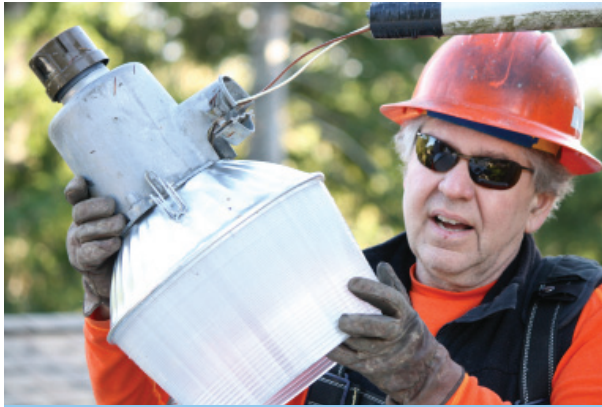
Figure 2. Mason PUD 3 lineman, John Donovan, replacing an old HPS area light with AreaMax. It's easy to see from these photos how the smaller and sleeker AreaMax housing.
