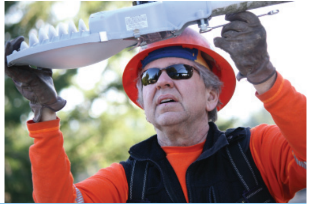
Figure 2. Mason PUD 3 lineman, John Donovan, replacing an old HPS area light with AreaMax. It's easy to see from these photos how the smaller and sleeker AreaMax housing.
